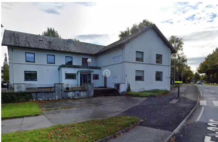
Jærveien 34 status 2021 (Foto Google Street View)
