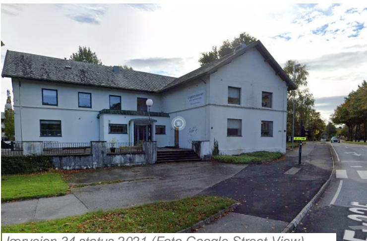
Jærveien 34 status 2021 (Foto Google Street View)
